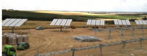
Commercial installation of our DACPV-280W25 in southern Europe. The nominal output per tracker is 13.4 kW
